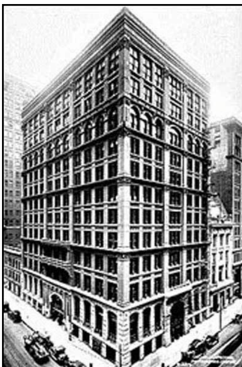
Home-insurance, 1885, (high building with steel) William Le Baron Jenney (engineer)
