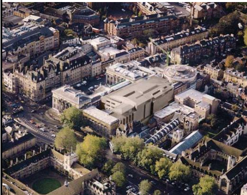
Aerial view of Ashmolean Museum, Oxford, by Cockerell, 1839-45
