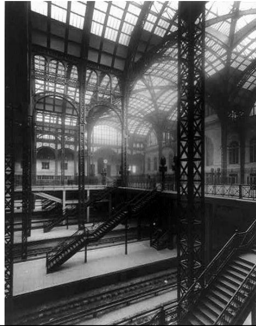
Interior view from the concourse level
