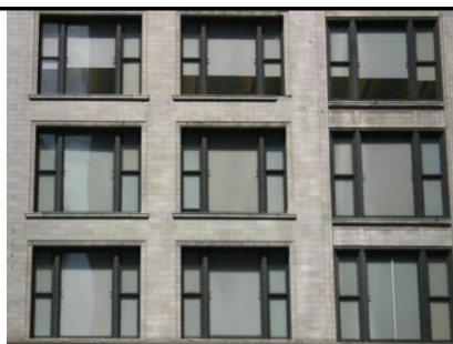
Chicago School window grid
